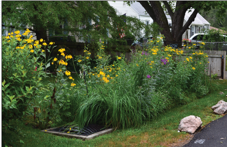
In a bioswale in Speedway, water pools and infiltrates in the landscaped basin (right side), which is lower than the left side, where the overflow drain receives excess runoff. The resident exemplifies the power of outreach. He has taken ownership of the plants installed in the right-of-way in his yard. Not only does he tend the plants, but he even painted the steel drain black so it will not rust.
